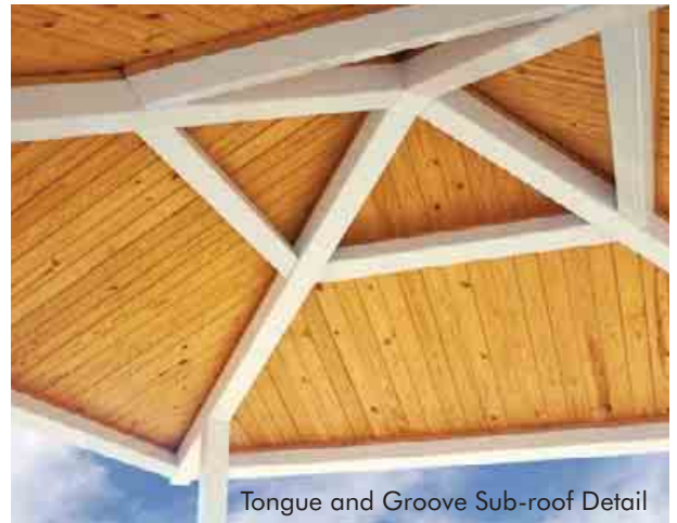
20' X 24' HIP RECTANGULAR SHELTER Shown with Square Columns & Timberland Blend Shingle Roof, 4:12 pitch (Tongue & Groove sub-roof shown).
